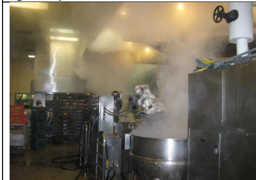
Figure 2. A photo of steam overflow around the hood
