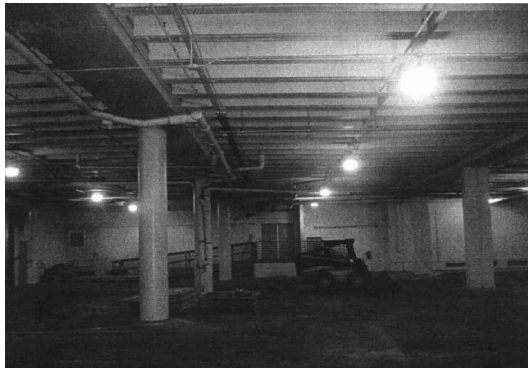
Figure 1. Photograph of garage ceiling area
